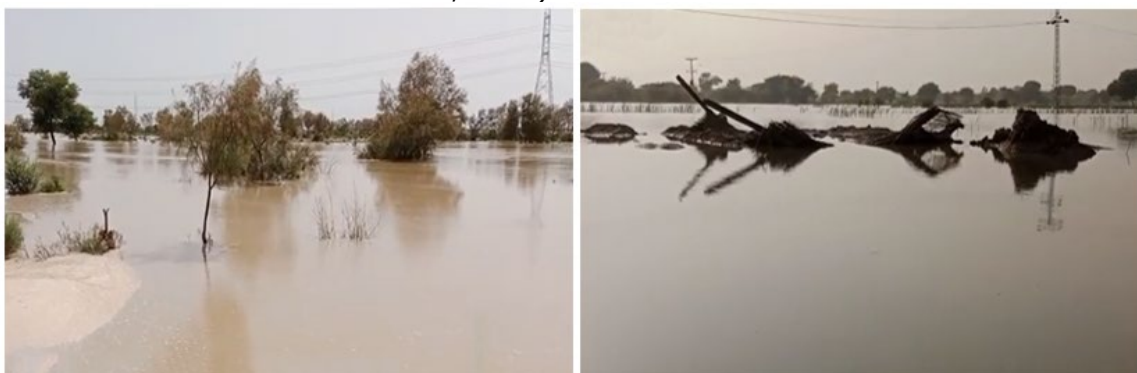
Figure 8. Impacts of the 2022 floods on physical infrastructure in the study area.
